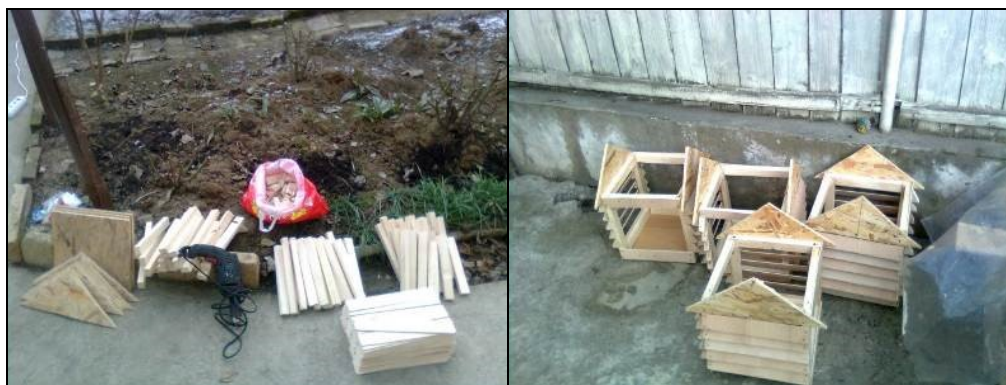
Fig. 3. Shelter materials (left) and shelter assembly (right)
